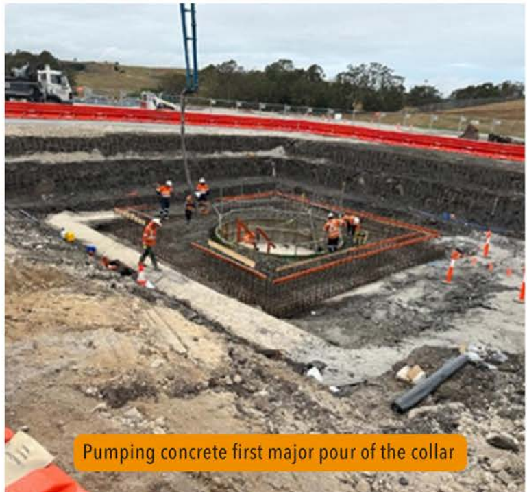
Blinding poured ready for syteel reo installation
