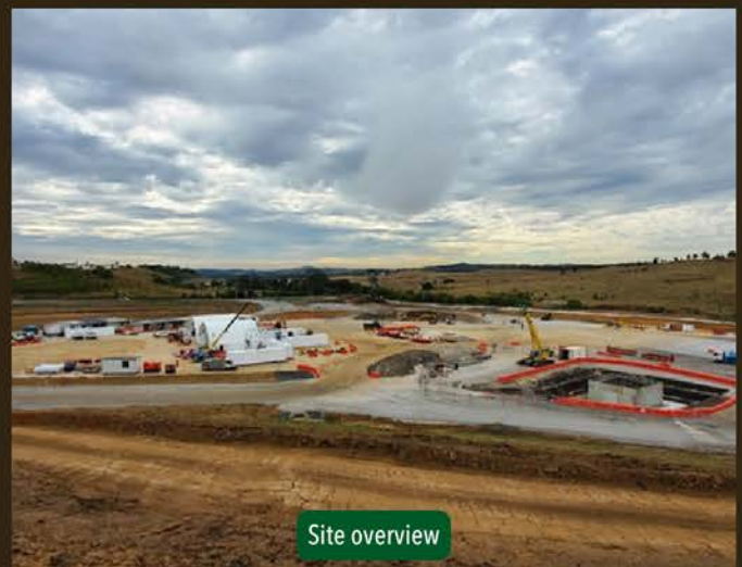
VS8 Collar Construction
