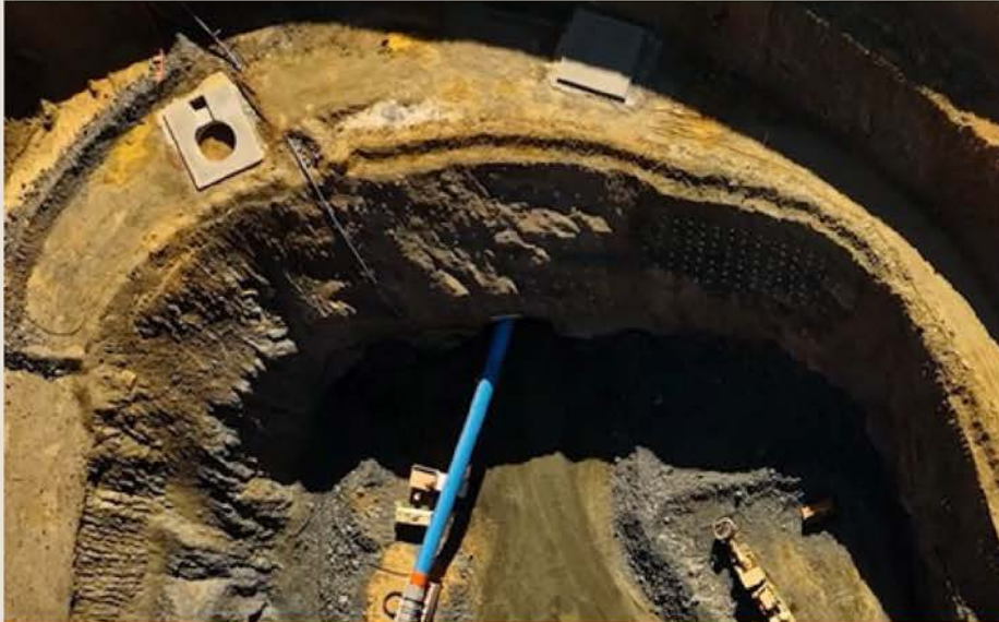
Overview of Portal, Fan, & Raise bore pads
