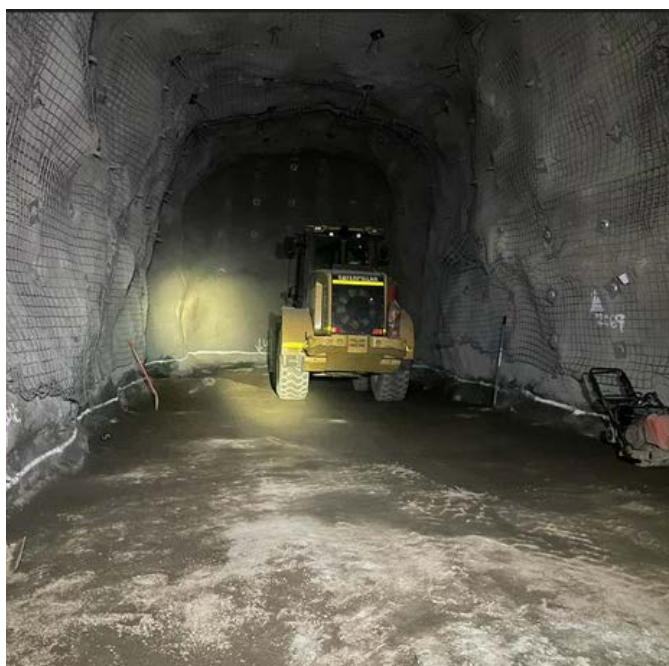
Wallaby Underground Workshop
